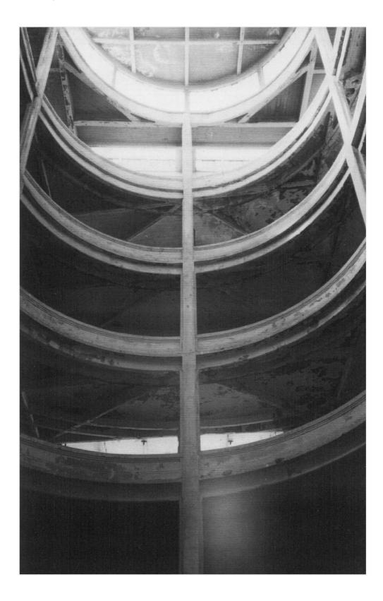
The metal press facility is all on one level while the office building is comprised of five above-ground floors with two spiral ramps at the far north and south ends of the complex, whose function is to facilitate the transport of items from one level to another.
