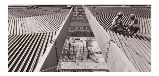
With his ferrocement "recipe," composed of layers of steel mesh filled with cement mortar that make it light, plastic and flexible, monumental domes, elegant barrel vaults, artistic crossed arches, futuristic spiral staircases are created.
